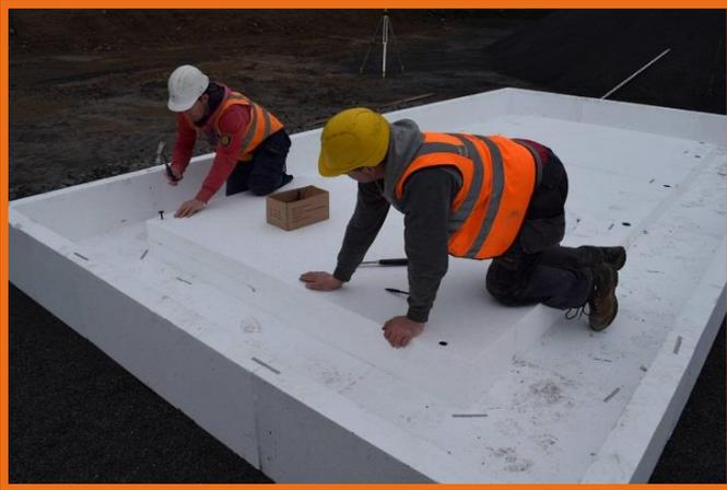
12. The second and subsequent layers of floor insulation are now installed, joints are staggered through the layers to prevent a continuous joint running from top to bottom. Plastic pins are provided to secure the sheets together. If not already in place DPC is fitted over the final layer of floor insulation and across the edge beam channel\*.
