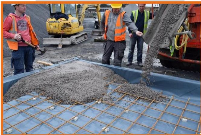
14. Prior to concrete placement a final check should be taken to ensure L sections are secured and if necessary further bracing applied, final levels are accurate across the floor area, reinforcement has been installed as per engineer's specification and all services are installed and secured.
