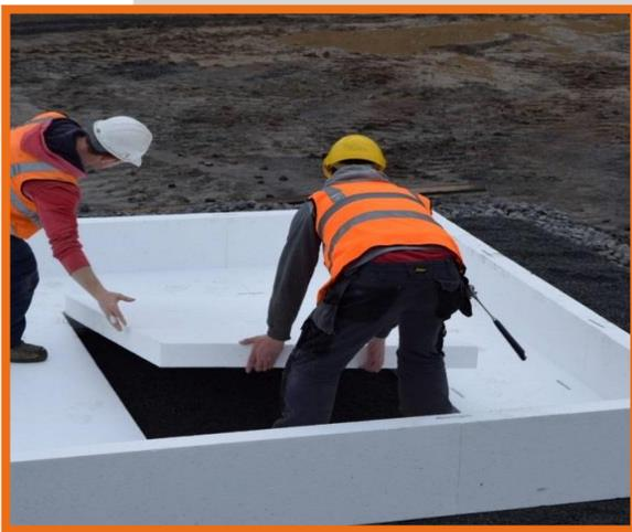
10. Placement of the first layer of underfloor EPS 100 sheets commences from the perimeter inwards.
