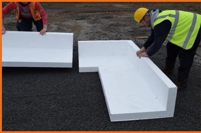
8. Starting from each corner L sections are set working in towards the wall centers, each component should be a tight fit to the next. L sections are supplied in fixed 2mtr lengths from the factory and may need to be trimmed on-site to fit the actual wall dimensions. Offcuts should be retained for future use. Steel combs are used to secure the L sections together and prevent movement.
